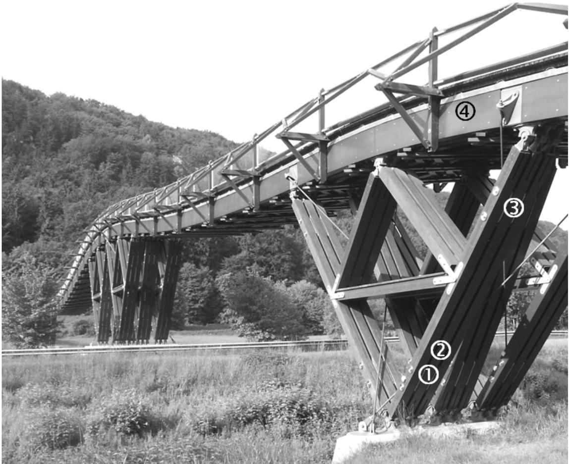
**Figure 7.3-3. Self-supporting pedestrian timber bridge in Essing, made from Norway spruce gluelam: ① Bottom nail plates, ② region above bottom nail plates for installation of measuring points remote from the nail plates, ③ upper nail plates, ④ main trusses covered with plywood.**
