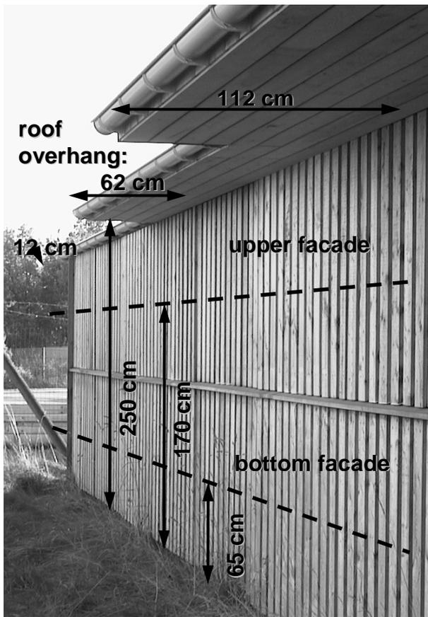
Figure 5: Board-on-board cladding with different roof overhangs in Tåstrup, Denmark. Dashed lines mark the heights of measurement points on the upper and bottom parts of the facade
