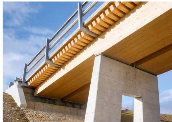
Figure 5: Timber road bridge Horen
