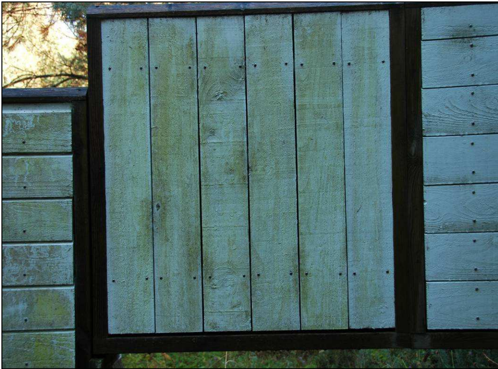
Figure 6.37 Differences in algal growth between panels SHCF (left), SVOF (centre) and SHOF (right). The latter panel had little growth whilst the other three painted panels were colonised by Desmococcus olivaceus over most of their surfaces.
