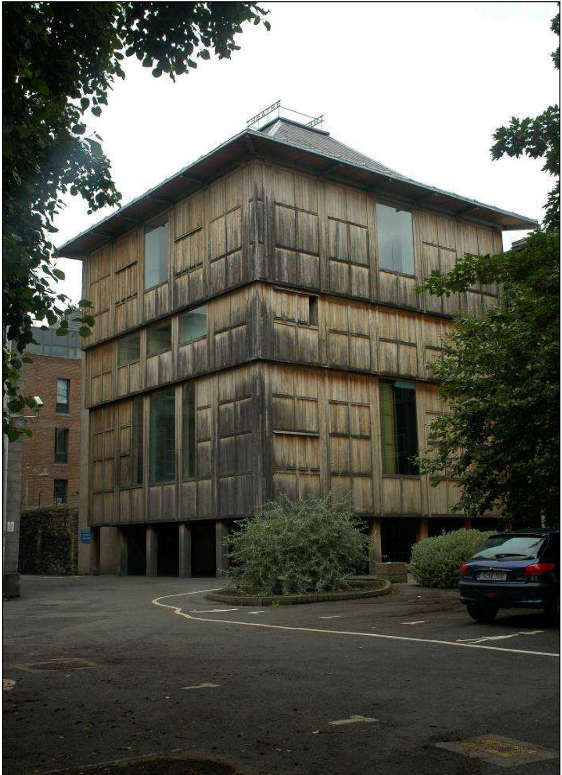
Figure 5.6 Celebration of moisture effects: the location and detailing of this timber clad building in Dublin has created a wide variation in microclimate conditions and correspondingly wide range of weathering effects. This was done in full knowledge of the likely consequences – it was an aesthetic decision. The timber was European oak ( Quercus spp.).
