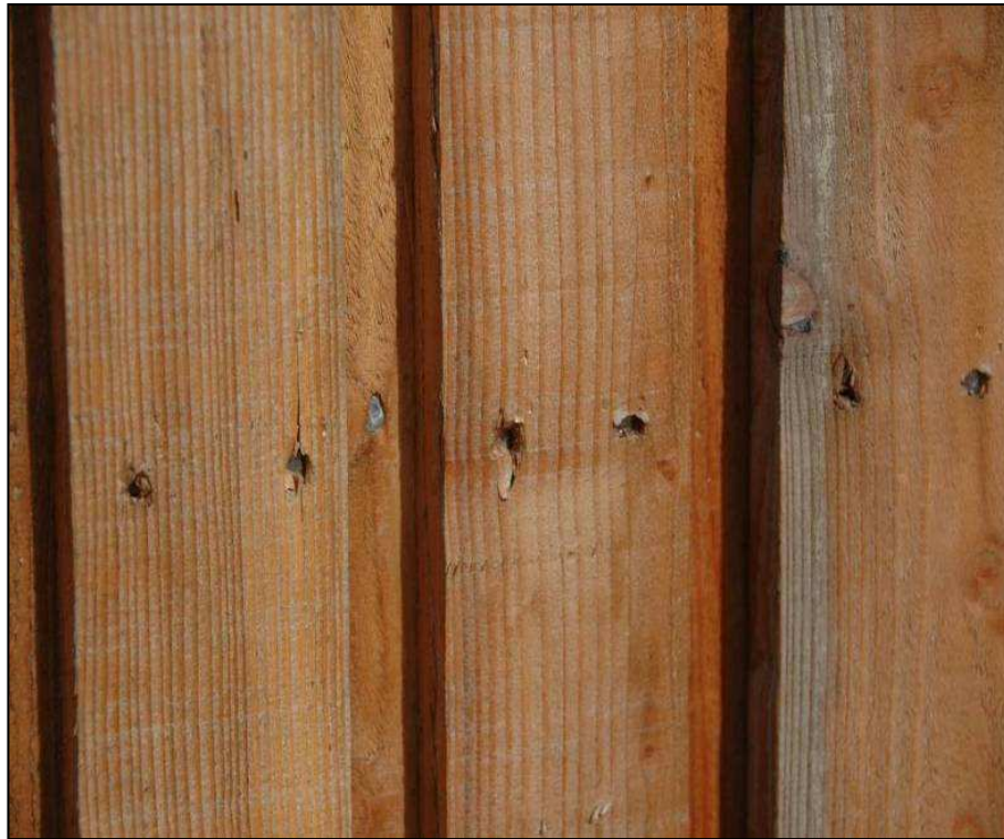
Figure A.2.5 These shot fired nails have been overdriven thereby creating water traps and splits.
