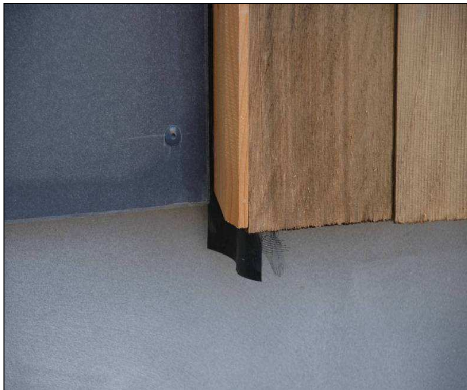
Figure A.2.12 A plastic DPC has been positioned between the cladding and vertical cavity barrier. Although essential with masonry cladding this detail is a potential water trap if used behind timber. Timber: preservative treated western red cedar.
