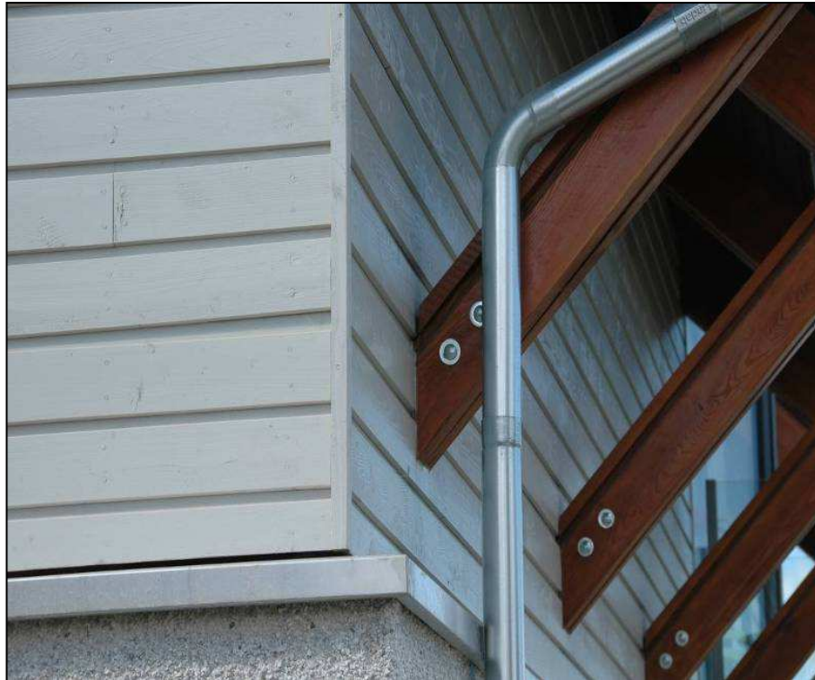
Figure A.2.17 These exposed structural timbers are butted against the cladding with a risk of water entrapment. Also the structural timber is local Douglas fir which offers little resistance against fungal decay.
