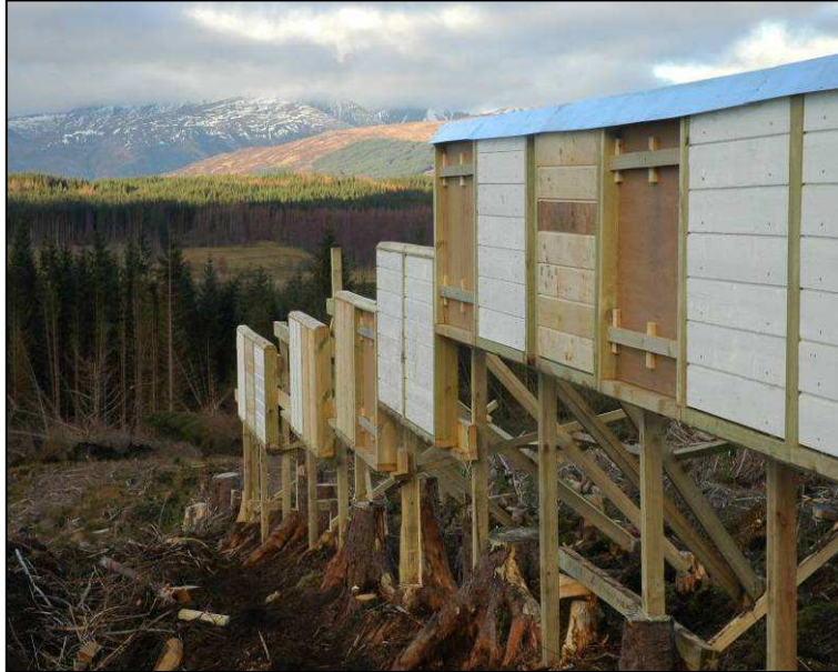
Figure 6.9 The Leanachan exposure site during construction
