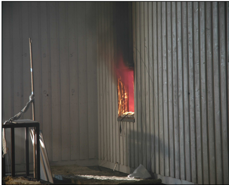
Figure 7.6 View of the facade just after flashover. The paint above the window has burnt off and the window frame is alight.
