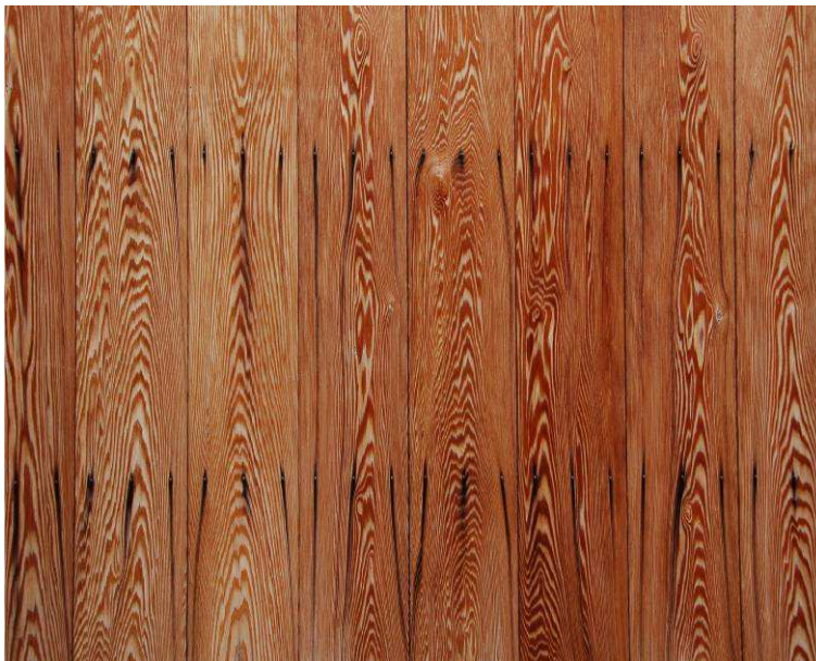
Figure 5.27 Iron-tannate staining due to crevice corrosion of ferrous fixings
