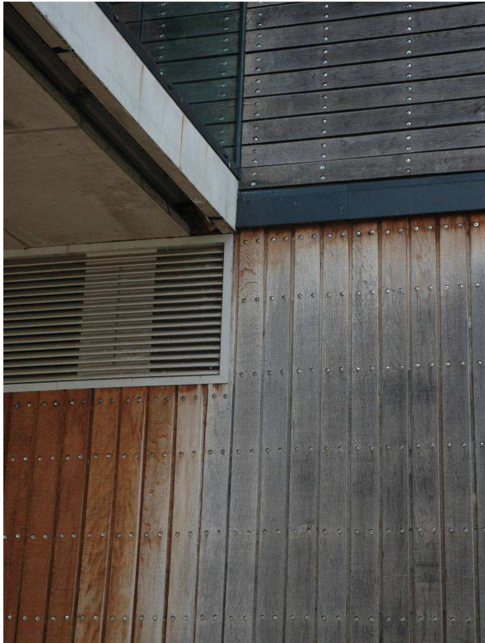
Figure 5.17 Weathering of timber is rarely uniform as it depends on a complex interaction of factors. This photograph shows cladding made of European oak ( Quercus spp.) at Henley River and Rowing Museum. On the bottom left the oxidised surface of the cladding has been protected from leaching by the projecting canopy. On the right side the cladding has been photo-degraded and the resultant breakdown products are, given sufficient moisture, supporting the growth of stain fungi turning the timber surface grey. All of the right hand side is equally exposed to UV light. The variation in grey staining appears to be due to differences in moisture availability affecting the growth rate of stain fungi.
