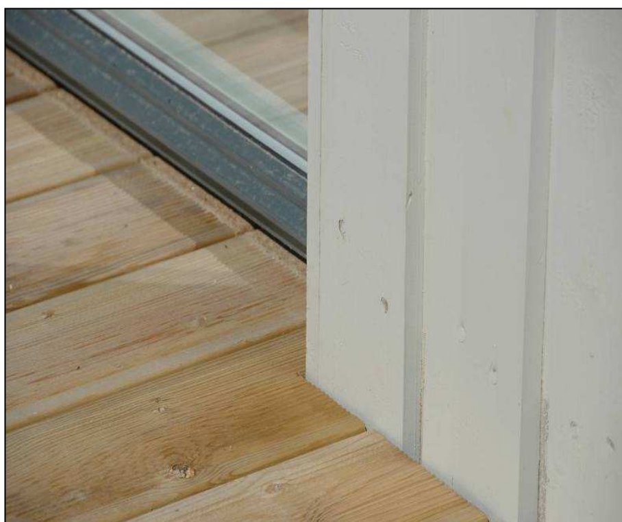
Figure A.2.10 Decking has been carried up to the wall, thereby creating a splashzone on the cladding (cladding timber unknown)
