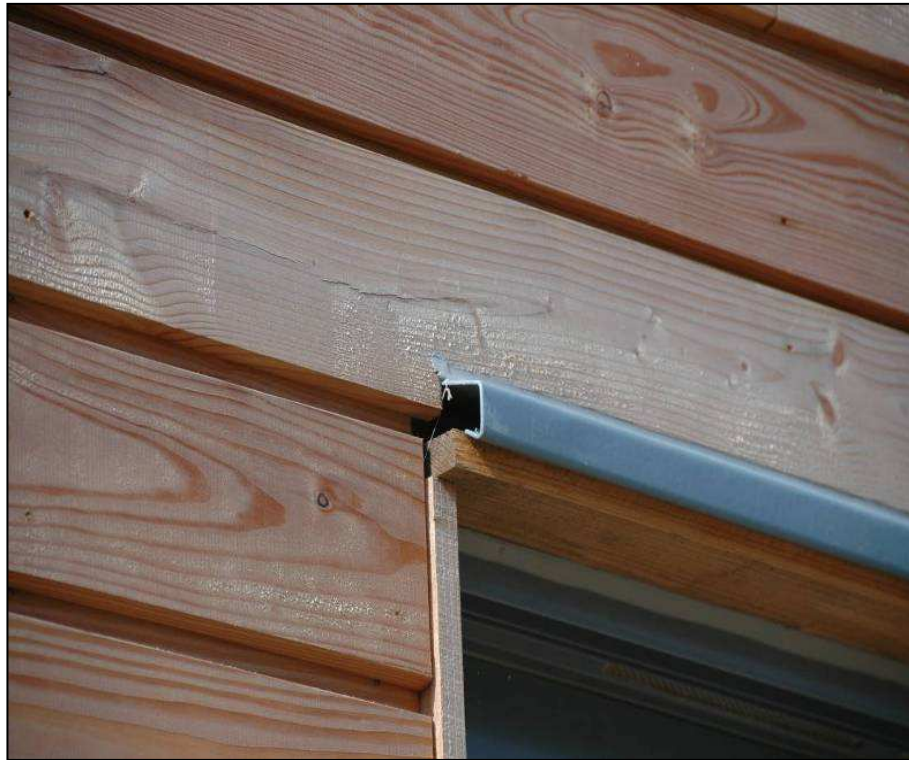
Figure A.2.3 Poor window installation. The flashing has been sealed with mastic thereby preventing cavity drainage and ventilation. There is no water bar at the end of the flashing. The space under the flashing will allow insects into the cavity.
