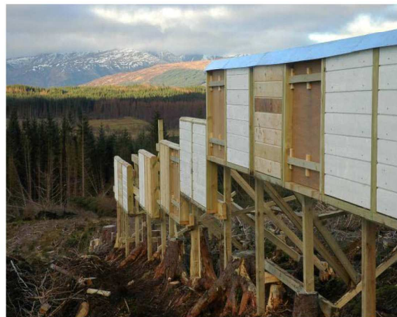
Fig 2. Part of the exposure trial during construction
