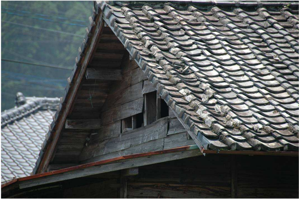
Figure 5.12 Thin cladding timbers are preferred in Mediterranean or sub-tropical climates. It is argued that they dry out quickly after wetting and thereby have a low decay risk. (Obi, Japan)
