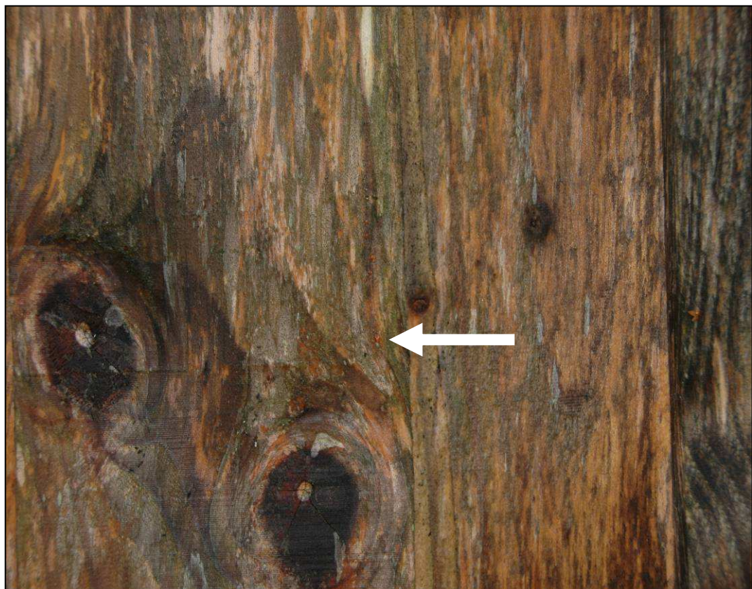
Figure 6.38 Widespread and unsightly surface staining along with occasional orange-red fruiting bodies (arrowed) of Dacrymyces stillatus .
