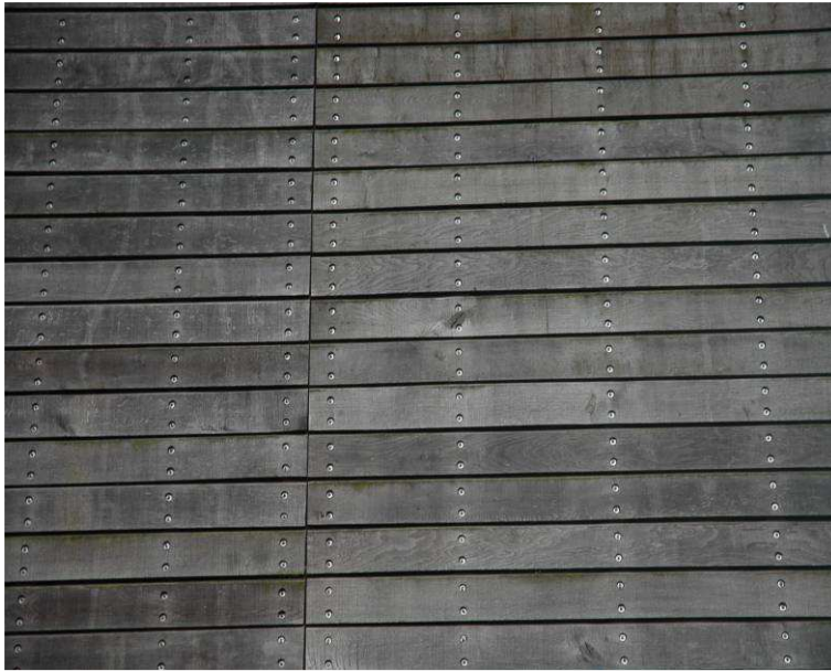
Figure 5.21 This oak cladding at Henley-on-Thames has stained in a uniform manner due to its sheltered humid site
