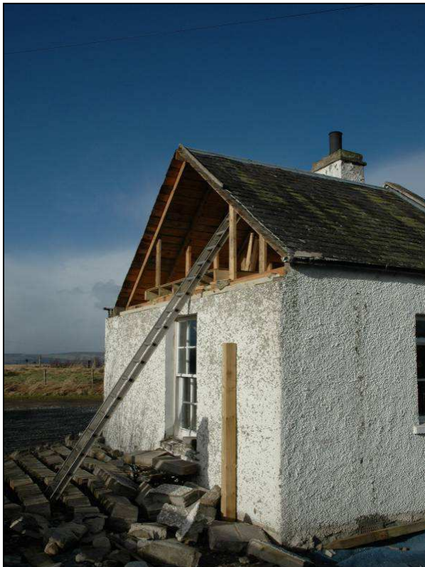
Figure 5.29 The masonry cladding on this gable near Inverness was inadequately fastened to the timber structure and so had little resistance to outward wind suction.
