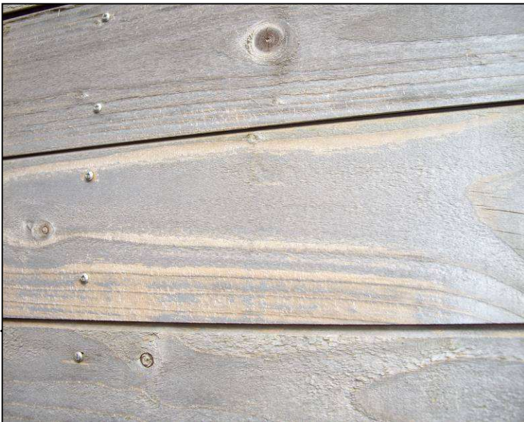
Figure 6.35 These stripes are due to wasps harvesting weathered timber.
