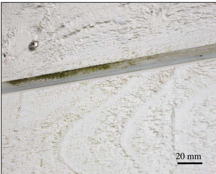
Figure 6.36 Algal growth on the bottom edge of a coated board.
