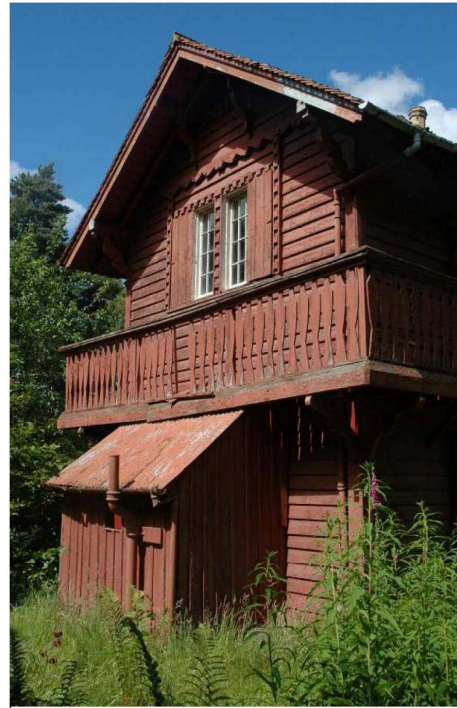
Fig 7. Most of this cottage was built in 1834 and has survived remarkably well even though the timber used was not durable, nor preservative treated. Other timber cladding in the area has failed in as little as 17 years.
