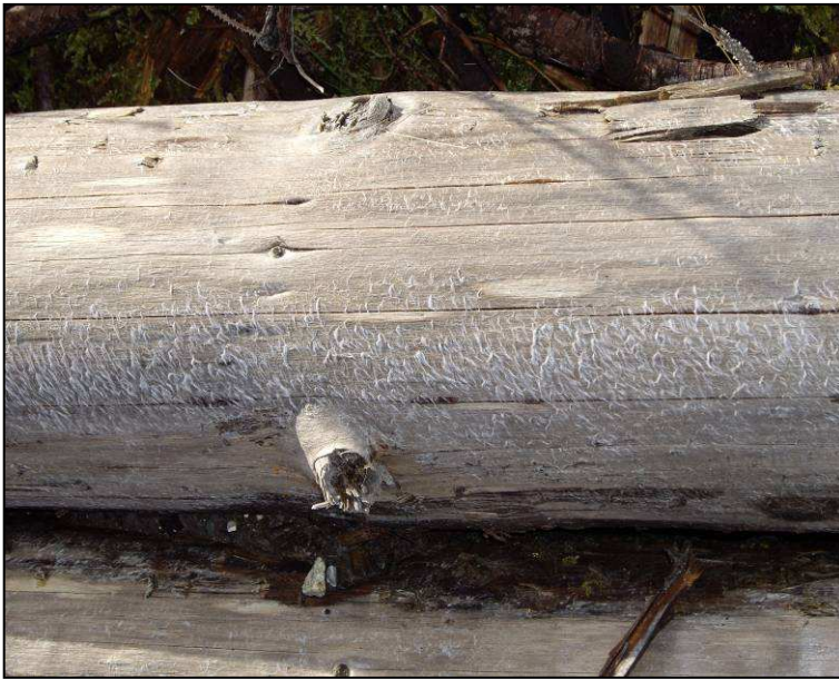
Figure 5.18 Fibres being exposed as the timber surface weathers.
