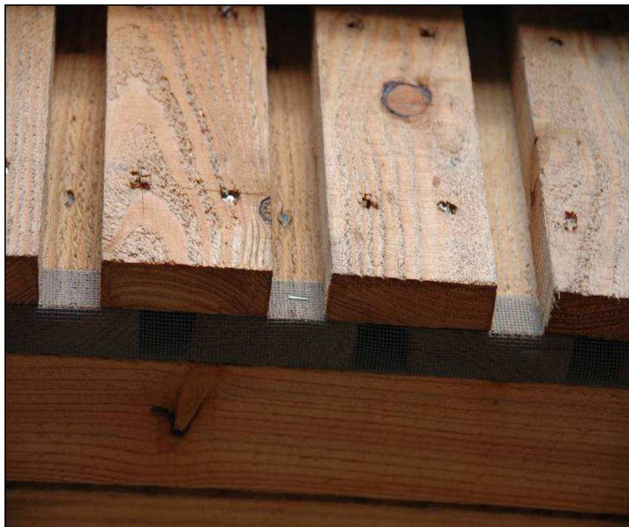
Figure A.2.8 These boards have been nail gunned together, thereby creating a risk of splitting the boards by preventing them from moving. Also note poor insect mesh installation and the over-driven nails.
