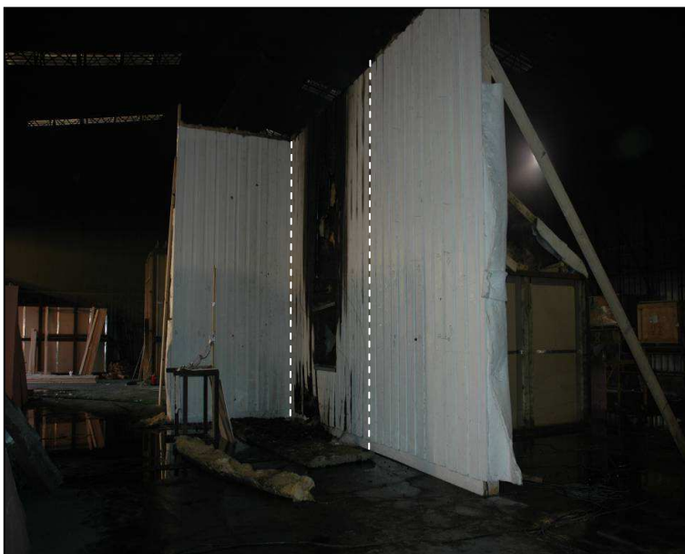
Figure 7.8 View of the facade after the fire was extinguished. Although the fire had spread the full height of the facade it had not spread laterally beyond the vertical cavity barriers (dashed lines).
