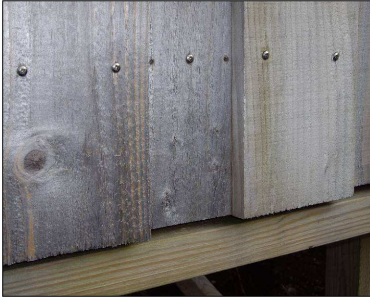
Figure 6.34 Weathering of uncoated timber, the heaviest staining is near the bottom of the boards.
