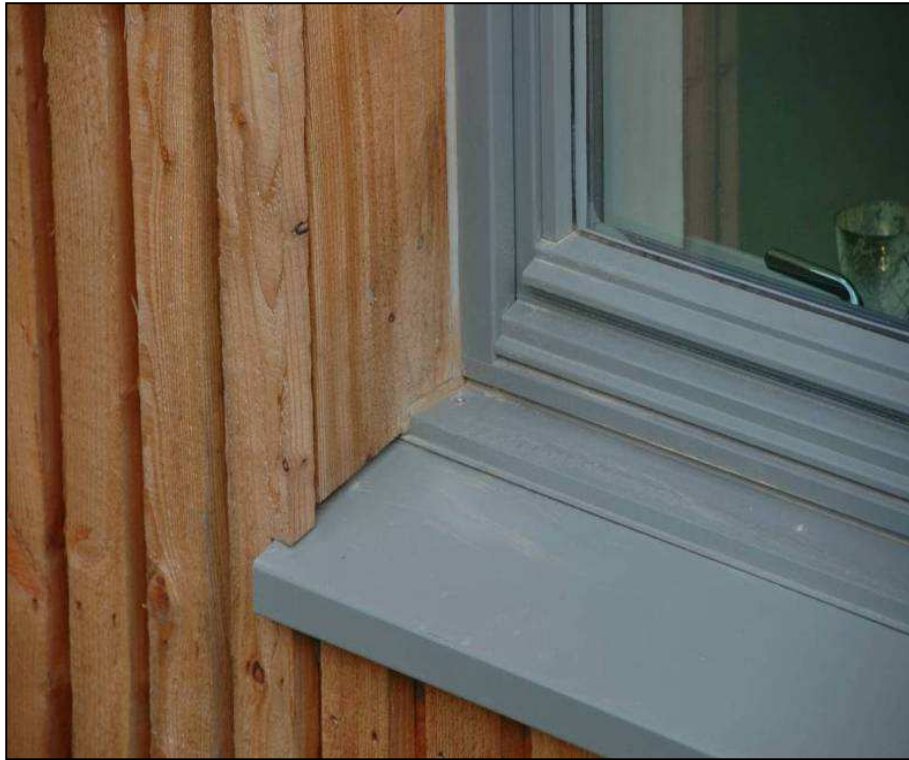
Figure A.2.1 Poor window installation. The lack of space below the boards ends will trap water, as will the mastic sealant. There is no water bar at the end of the metal sub-sill flashing.
