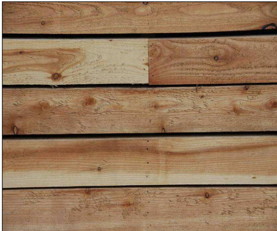
Figure A.2.14 The light coloured areas are sapwood, this should have been graded out. Also note the use of lost head nails.
