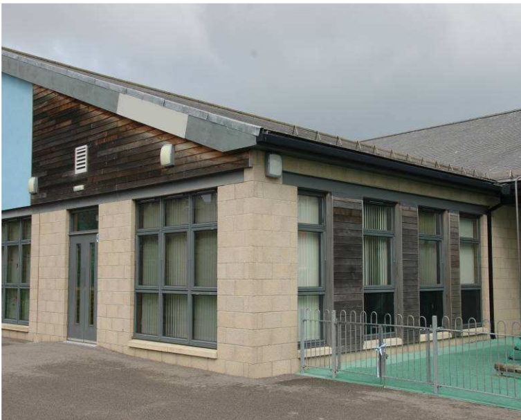
Figure 5.22 This western red cedar cladding in Aberdeenshire has been exposed to wind-driven rain at the gable while the three side panels have been sheltered. This variation in wetting has resulted in marked differences in fungal staining.
