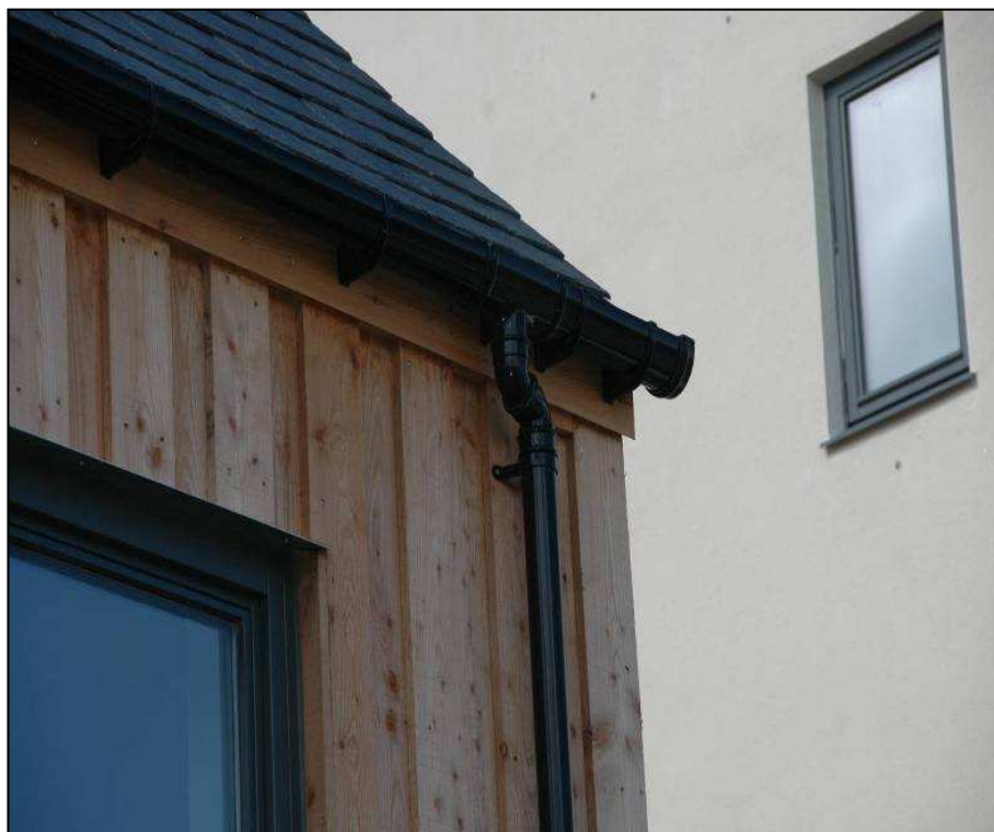
Figure A.2.9 No eaves ventilation.
