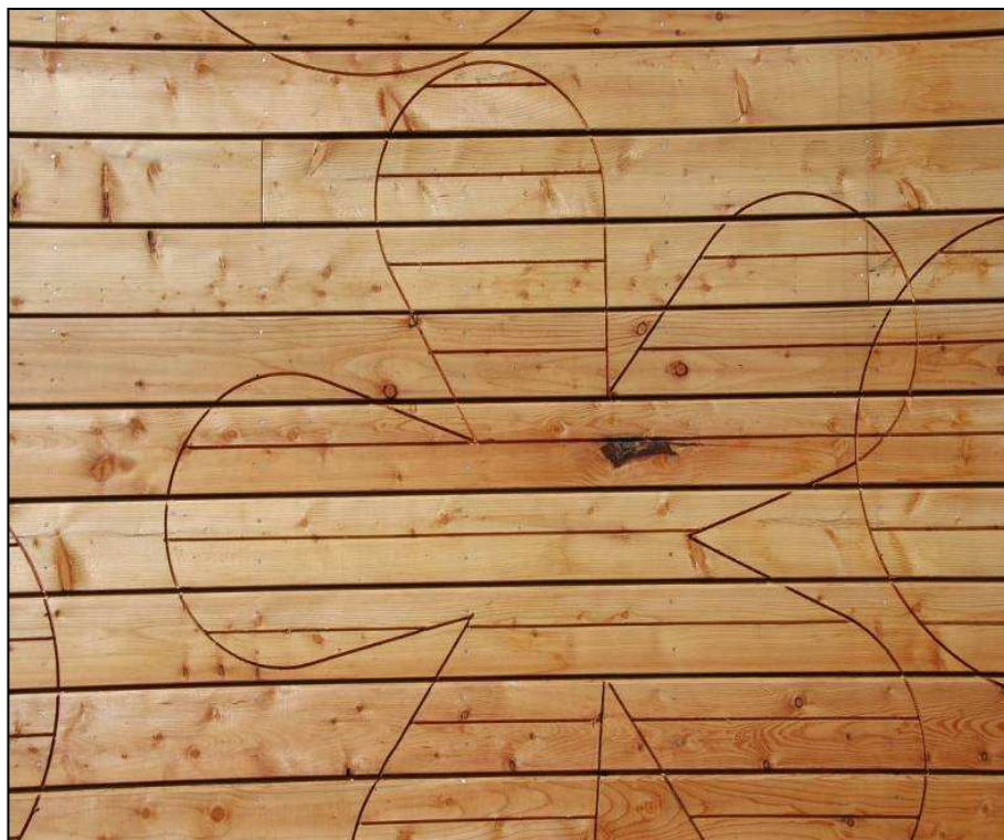
Figure A.2.18 This pattern has been routed into the timber using a simple rectangular cutter profile. Every routed line has horizontal edges that will trap water.
