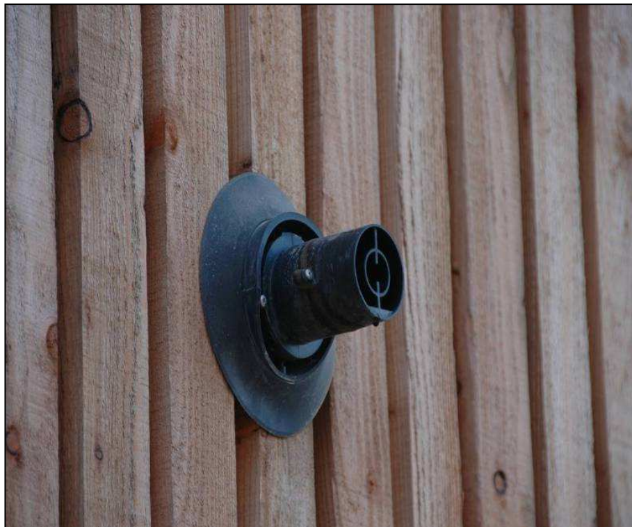
Figure A.2.6 This duct cover is only suitable for use with masonry cladding. It has created a water trap when used with timber.
