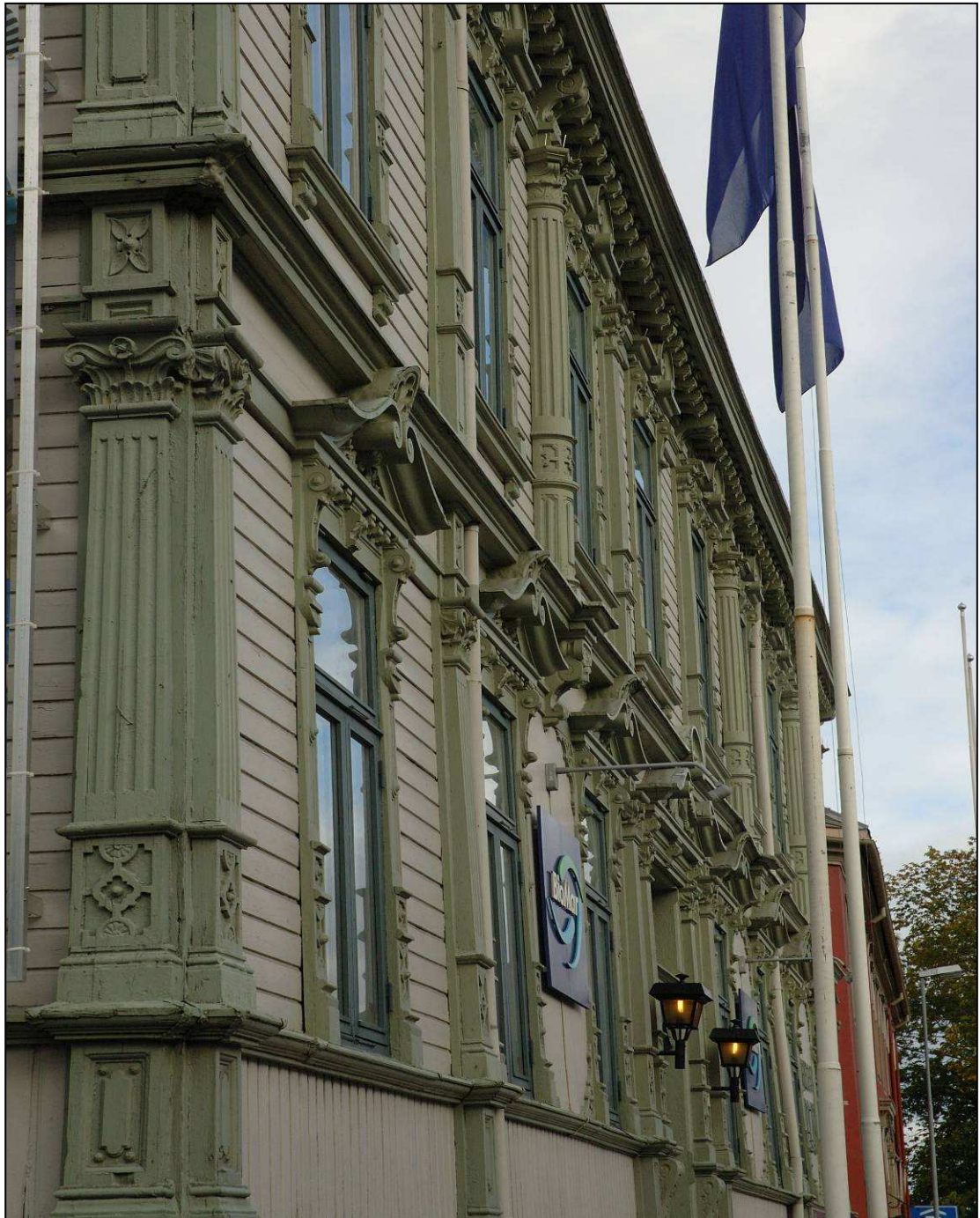
Figure 1.1 Late 19 th century timber cladding in Trondheim, Norway. Similar facades are found in most towns in western Norway; they were constructed using untreated European whitewood and redwood ( Picea abies and Pinus sylvestris ) These facades illustrate that durability class 3 to 5 timber in combination with elaborate detailing can achieve a long service life providing it is designed for durability and regularly maintained. Key measures include metal flashings on all horizontal projections, the avoidance of water traps, an opaque surface coating with fungicidal protection and the rapid replacement of any component that fails.
