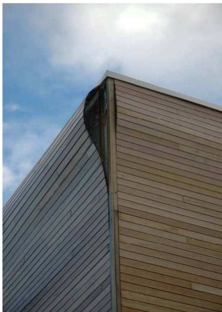
Fig 1. Failure of timber cladding due to inadequate movement provision
