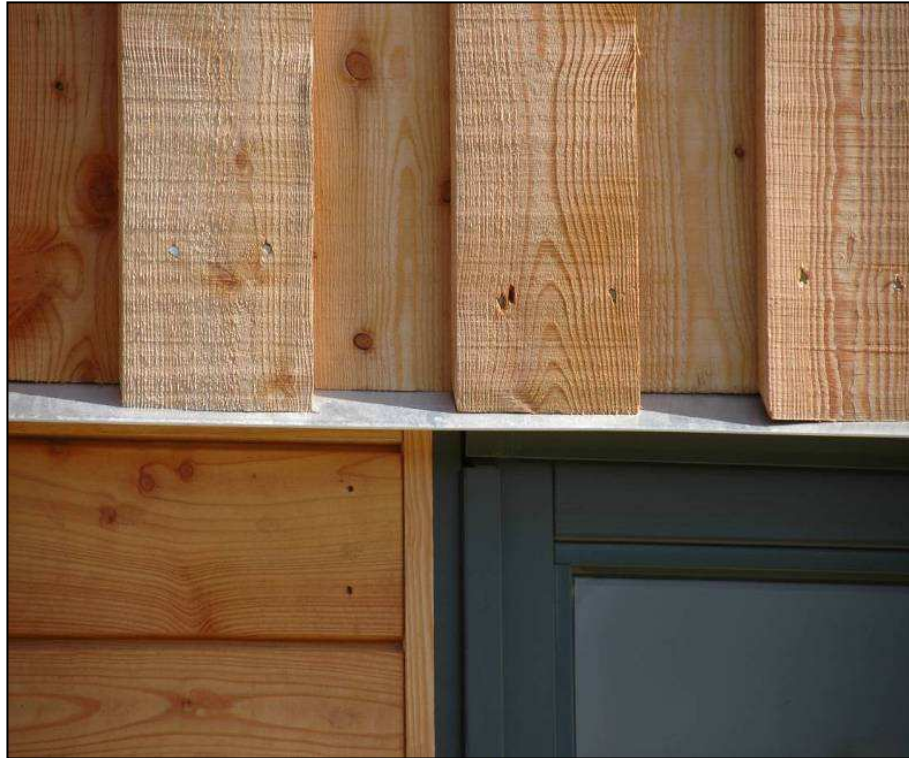
Figure A.2.15 These boards have been butted against a flashing thereby creating a water-trap as well as blocking off cavity ventilation.
