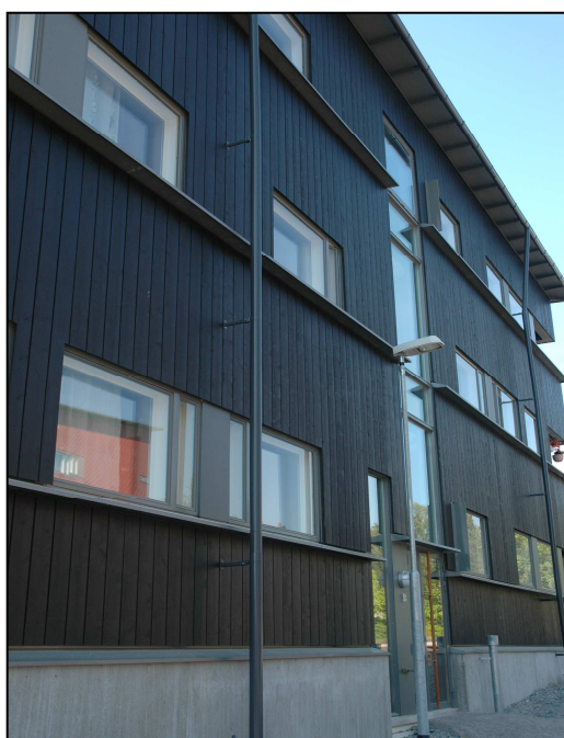
Figure 7.2 Horizontal flame deflectors used to slow external flame spread on a timber-clad block of flats in Porvoo, Finland.
