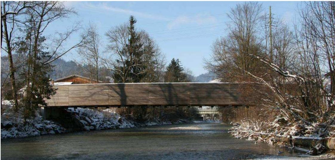
Figure 1. Timber traffic bridge in Obermatt
