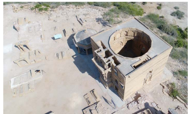
Figure 5. The highly significant tomb of Jam Nizam Al Din at the north end of the Makli Hills, World Heritage property
