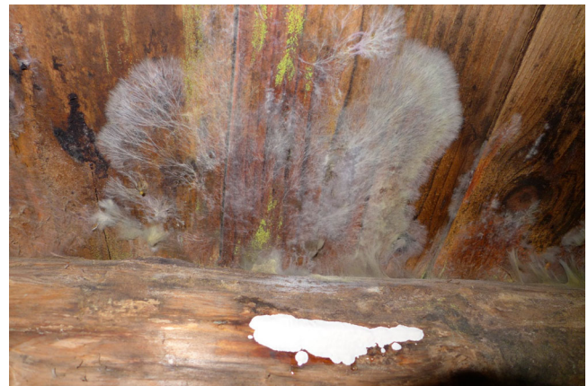
Figure 3. Mycelia of Antrodia sp. growing on the surface of wood in the cellar.
