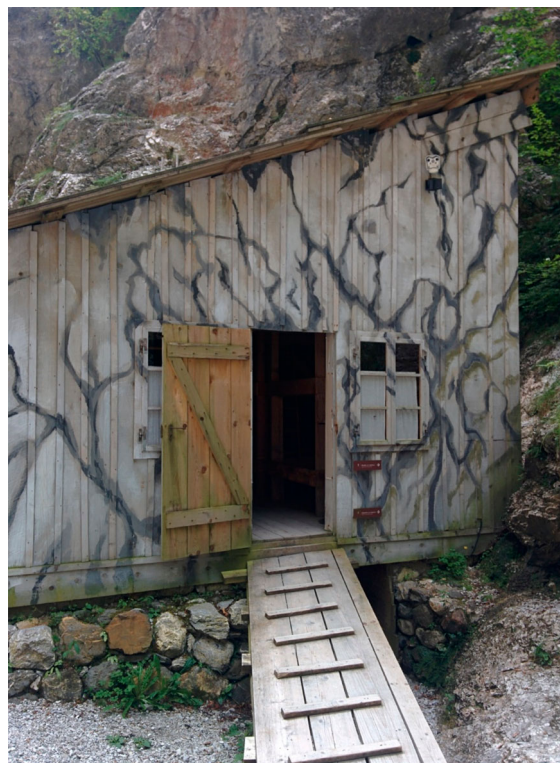
Figure 1. Cabin for the wounded at the WWII partisan hospital franja. Measurements were performed in the cellar (bunker) below the cabin, on the façade facing the hill, and on the first floor.
