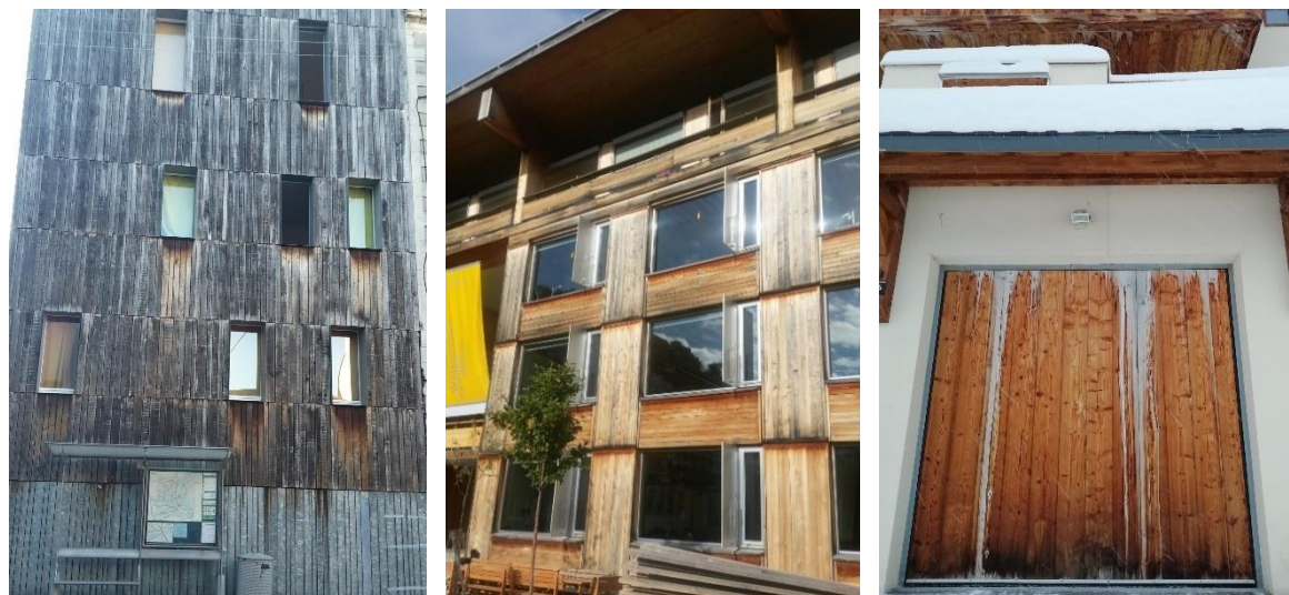
Figure 3: Facades with horizontal and vertical wood grain alignment in (left to right) Nantes, Biel and Les Menuires
