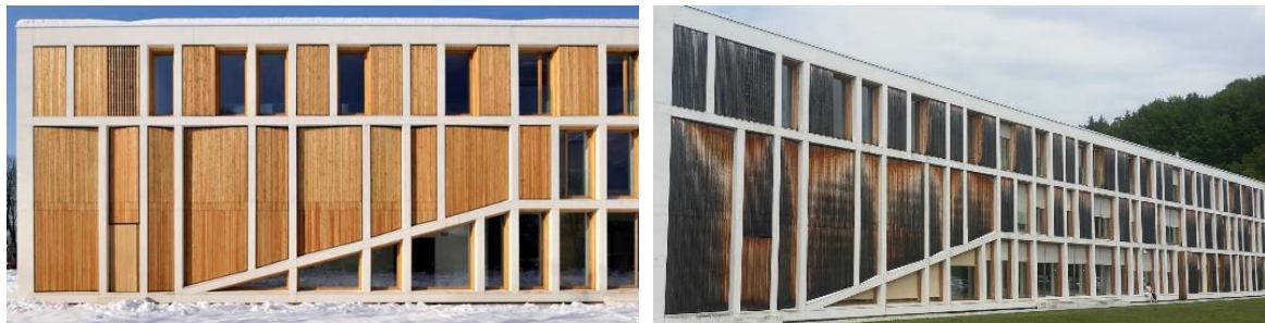
Figure 1: Façade of the Biotechnical faculty of the University of Ljubljana shortly after construction (Source: https://www.e-architect.com/images/stories/slovenia/biotechnical_faculty_ljubljana_k260510_m4tb.jpg ) (left) and after 8 years of exposure (right)
