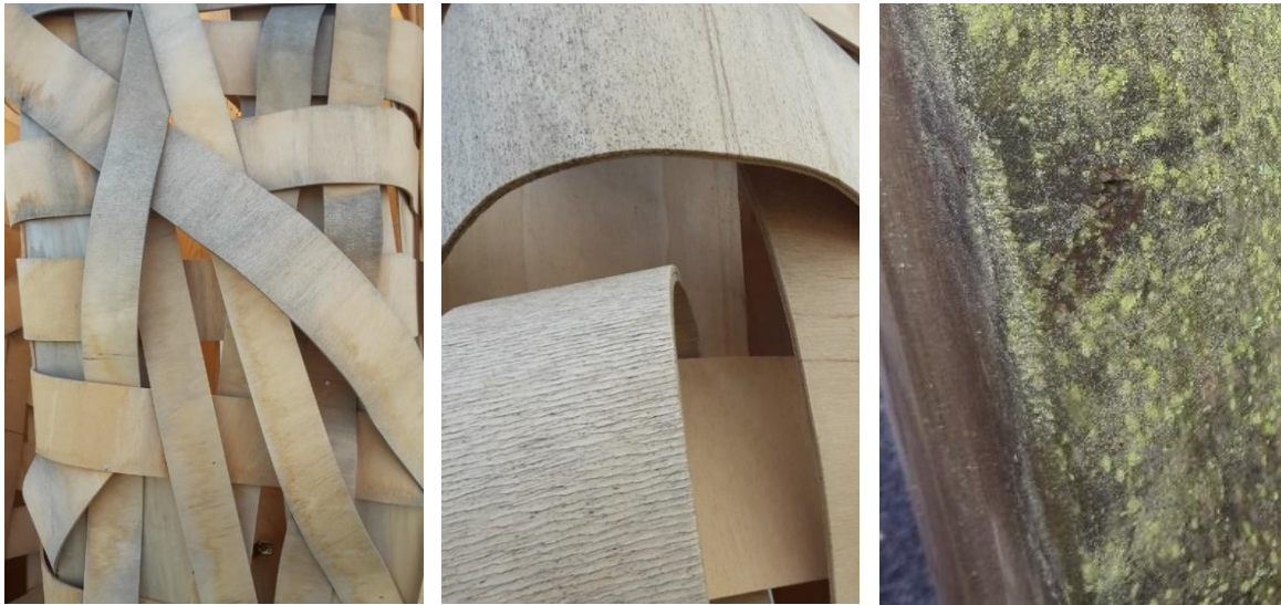
Figure 4: Wood exposed and attacked by fungi, visible to the naked eye
