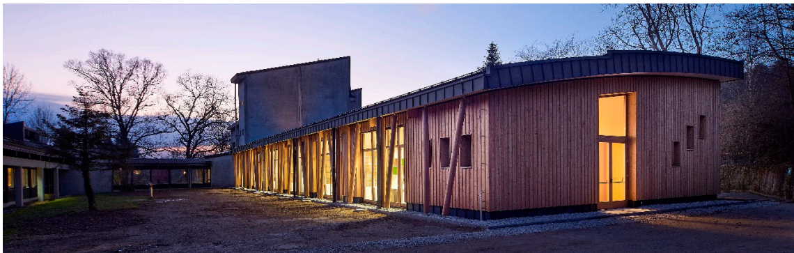
Figure 1. Annex to the existing building of the Department of Wood Science and Technology in Ljubljana (photo: Damjan Švarc).
